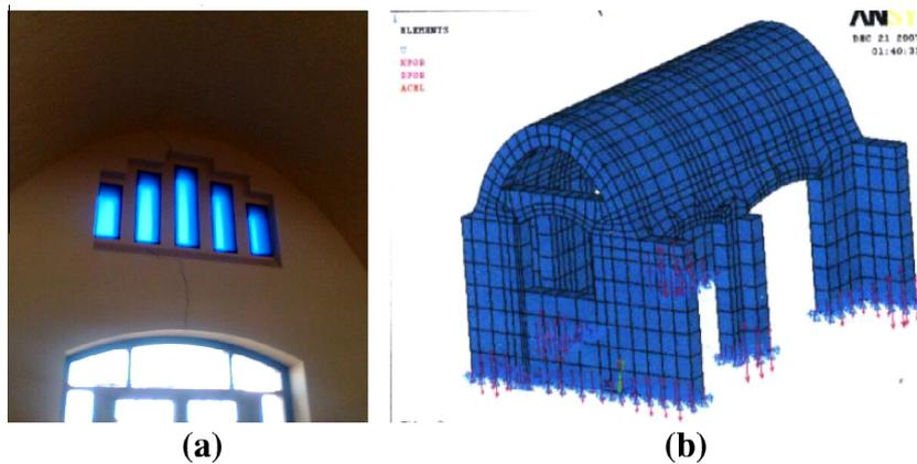
Fig. 15 The observed crack and the finite element mesh for vault.
