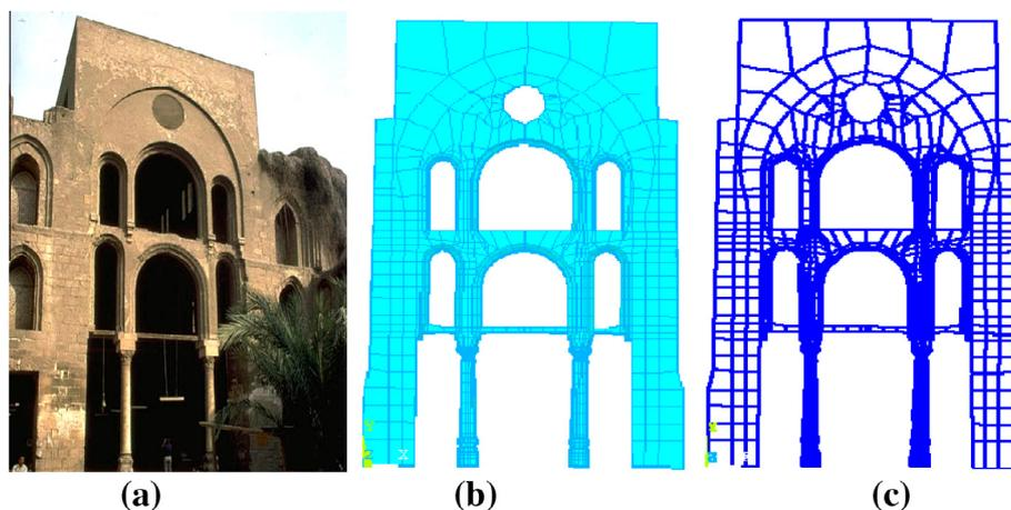
Fig. 12 Qalawon Madrassa; (a) interior facade, (b) nonlinear analysis model and (c) crack pattern.
