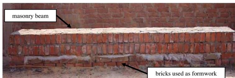
Fig. 7 The finished masonry beam A.
